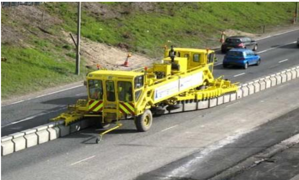
Quick Movable Barrier on test
